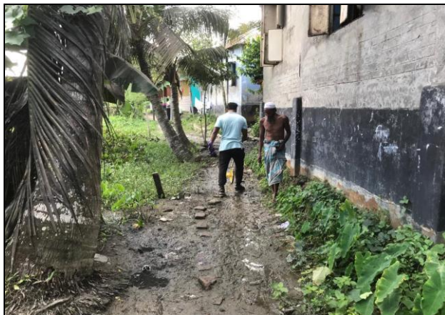
Drain-025, Hossainpur Paurashava
