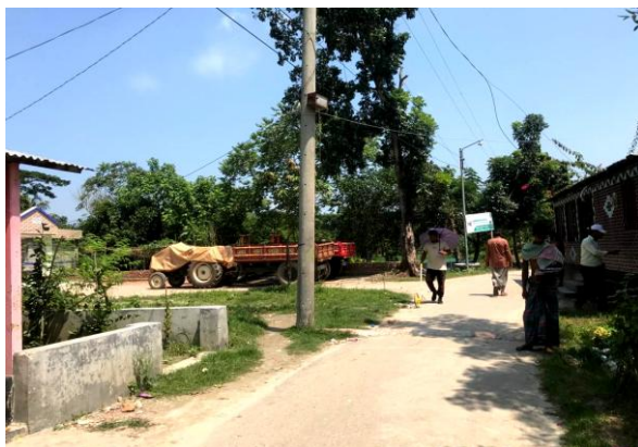
Drain-007, Hossainpur Paurashava
