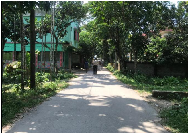
Drain-024, Hossainpur Paurashava
